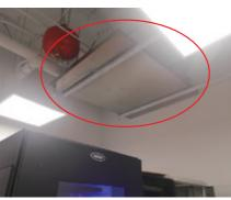
Cover around piping with waterproof material Trays installed for double protection
